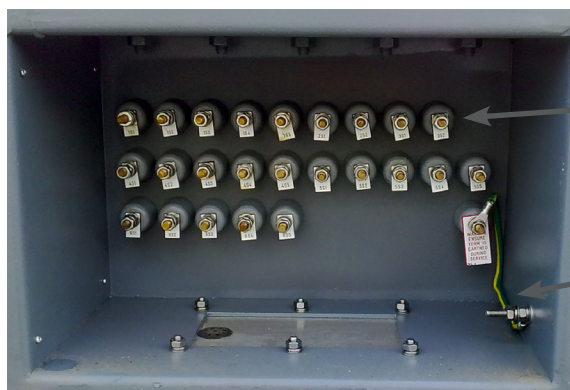
Capacitively Graded Screen External Earth Connection
